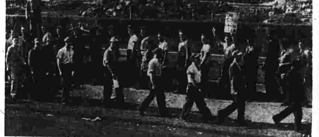
CIO pickets parade outside the Federal Shipbuilding and Dry Dock Company yards at Kearny, N. J., in a walkout of 16,000 units which halted production on $403,000,000 worth of Naval and merchant ships. In the background at left are Naval vessels under construction.
